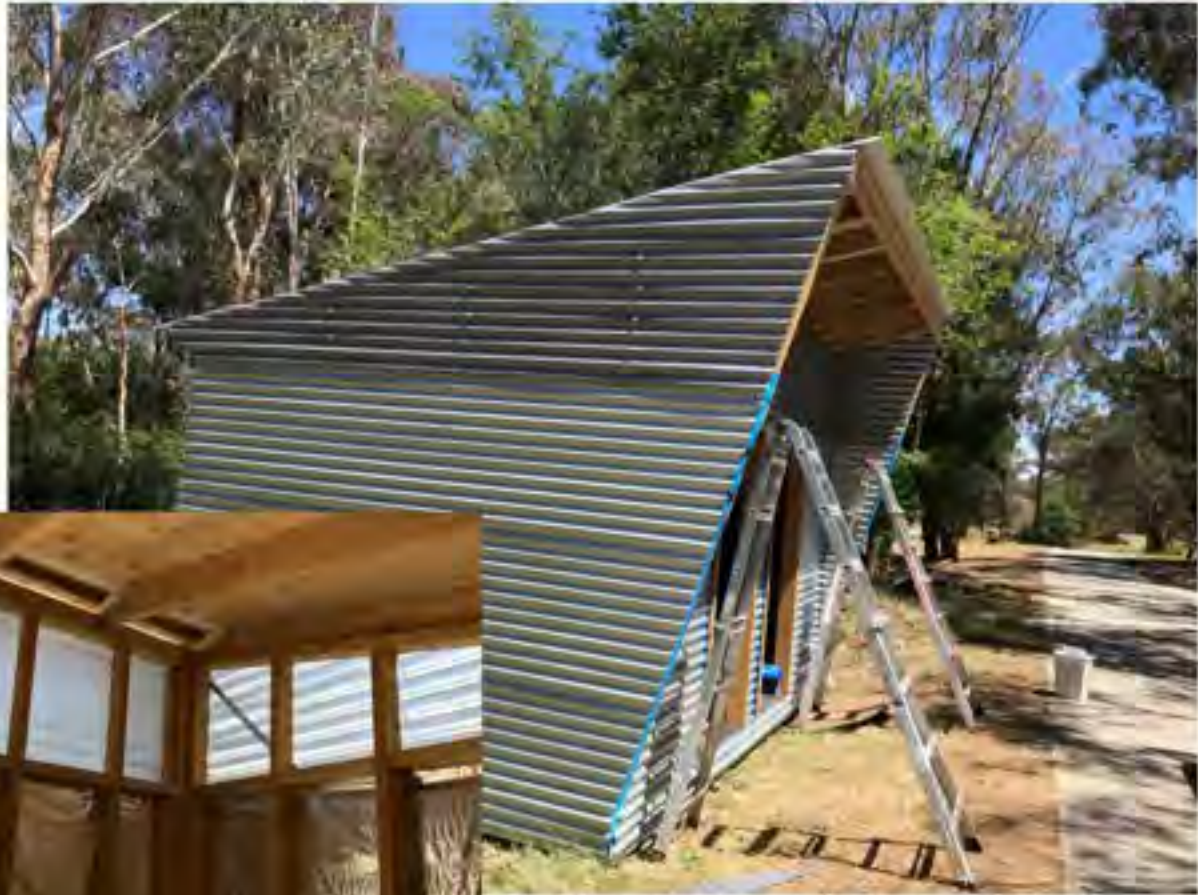
Cladding completed, flashing yet to be fitted. Inset: Clever use of polycarbonate sheeting to allow natural light in.
