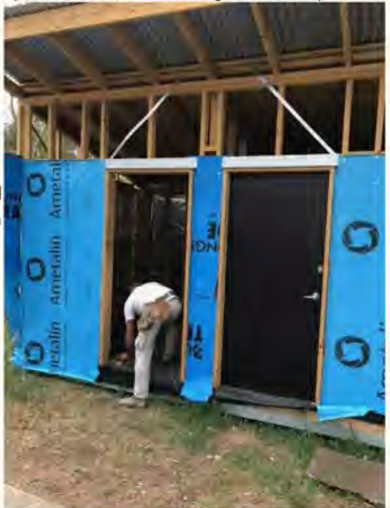
Right hand door hung, left hand door receiving David's expert attention to perfect the fit.
