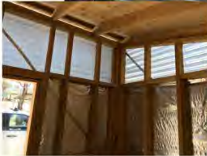
Cladding completed, flashing yet to be fitted. Inset: Clever use of polycarbonate sheeting to allow natural light in.
